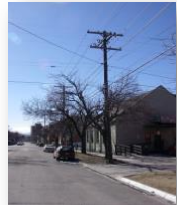
Figure 19 Utility – tree conflict
